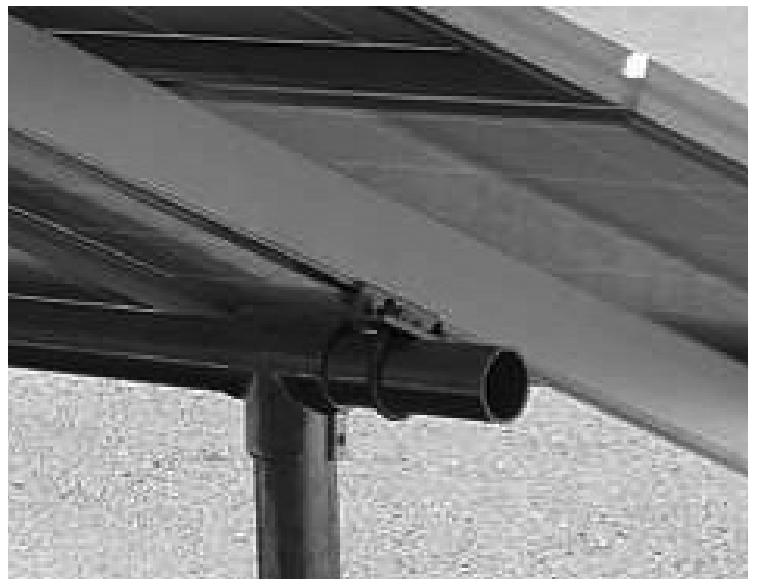
Attach Pipe Mount to Rail
